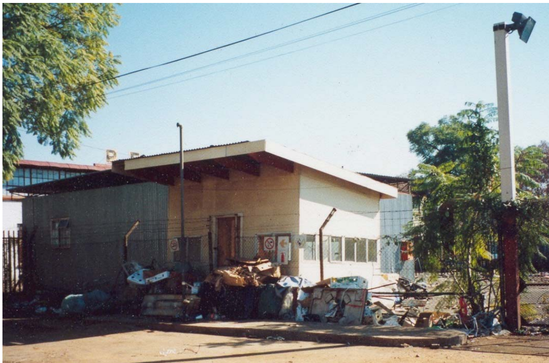
Figure 3: Derelict buildings impact negatively on the neighbourhood and can increase the fear of crime
